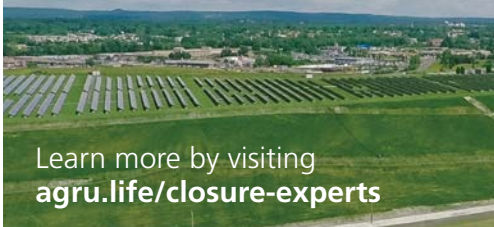
35 acre landfill closure in Connecticut, topped with 5 acre solar array.
